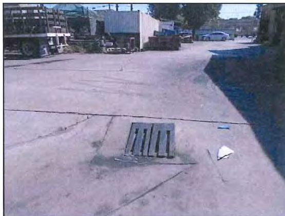
Photo #15: Run-off drain in yard area.
