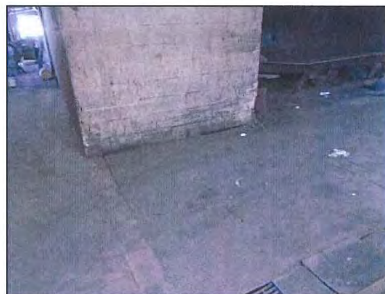
Photo #6: Steel plate near processing area.
