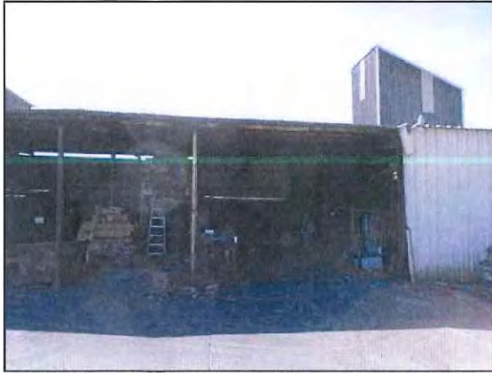
Photo #13: Exterior metal recycling receiving area.
