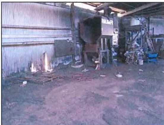
Photo #9: General interior conditions at Subject Site, blackened sand material noted on floor.
