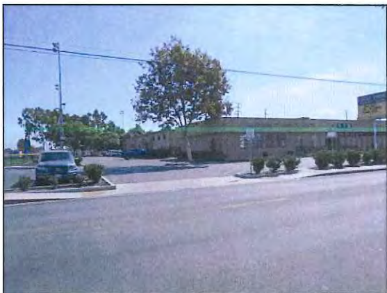
Photo #19: Surrounding properties, viewed east across Otis Avenue.
