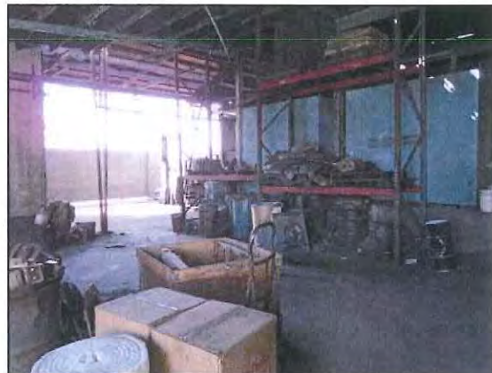
Photo #11: General interior conditions at Subject Site.
